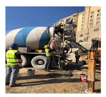
The inclusion of Xypex's active ingredients in the concrete enables ongoing crystal generation in the presence of moisture, ensuring sustained water-proofing. This application of Xypex products under-scores their capability to deliver durable and long-lasting below-grade waterproofing solutions.
